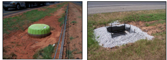
SRD Protecting Inlet
