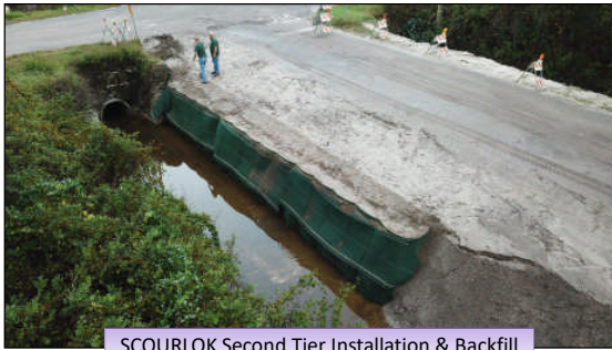
SCOURLOK Second Tier Installation & Backfill
