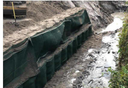
Reconstructing Roadway Shoulder Above SCOURLOK
