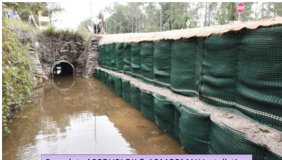
Completed SCOURLOK & ARMORMAX Installation
