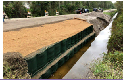
Topsoil, Seed & Erosion Control Blanket Placed on Top of ARMORMAX for Roadway Shoulder Vegetation Stabilization
