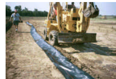
Once the (1) fabric is sliced into the soil, (2) compact,
