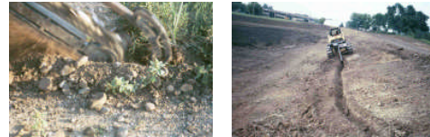
Traditional Trenching Works, But Requires Careful Attention to Detail
