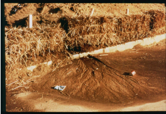
Typical straw bale installation (failure)
