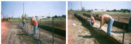
(5) Install posts, (6) tie up fabric
