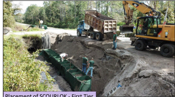
Placement of SCOURLOK - First Tier
