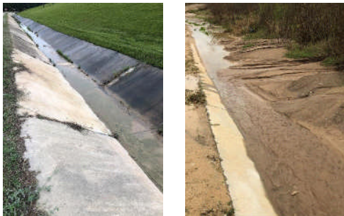
Perimeter Channels of ClosureTurf Versus Soil Cover (Photos taken on Nov. 2018)
