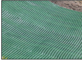
TRMs have primarily polymer structures
