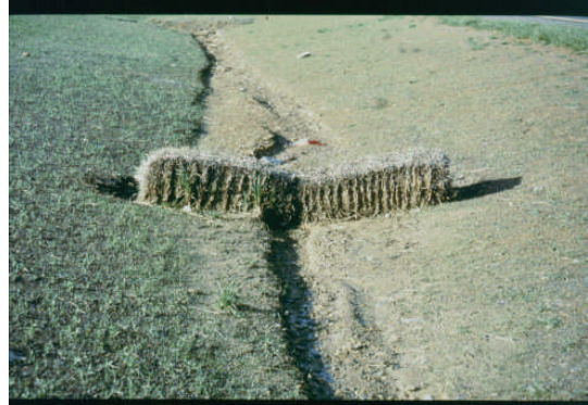
Typical straw bale installation (failure)
