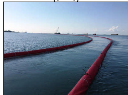
Geotube Turbidity Curtain
