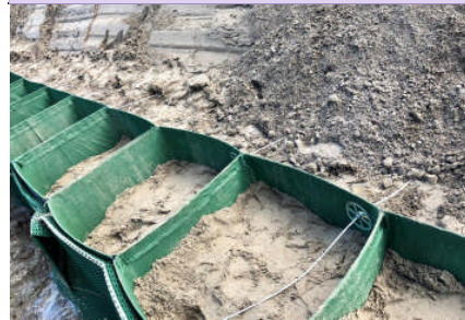
Cell Fill, Unit Backfill and Engineered Earth Anchors
