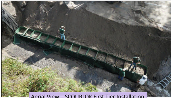
Aerial View – SCOURLOK First Tier Installation
