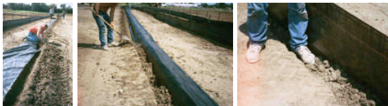
Once the (1) trench is dug, (2) place the fabric, (3) backfill, (4) compact,
