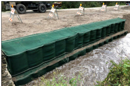
SCOURLOK & Roadway Shoulder Completion. Water Flow Restored to Canal.
