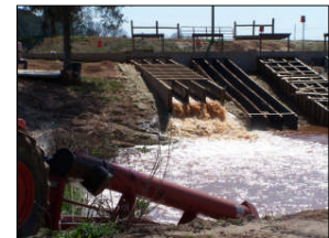
Long-term Flows are Facilitated by Pumped Recirculation
