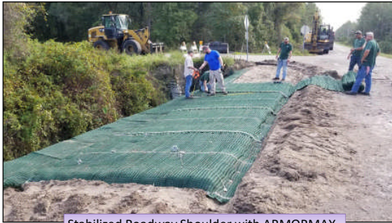
Stabilized Roadway Shoulder with ARMORMAX.
