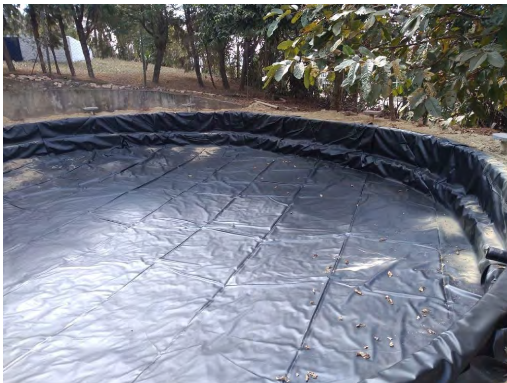
Figure 5: Circular tank coated with PVC geomembrane
