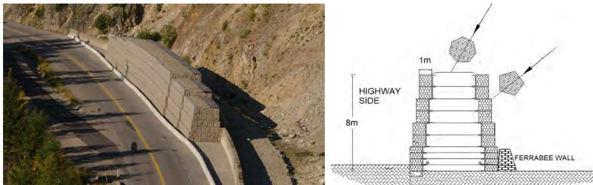
Figure 2. Rockfall protection embankment along the Trans-Canada highway. General view and cross-section (adapted from Simons et al., 2010).
