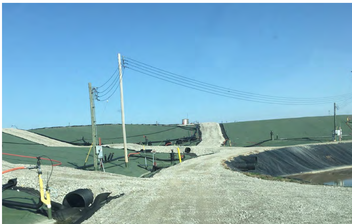
Figure 7 – Roads Overlying an EGC Used for Anchorage and O & M Access Activities
