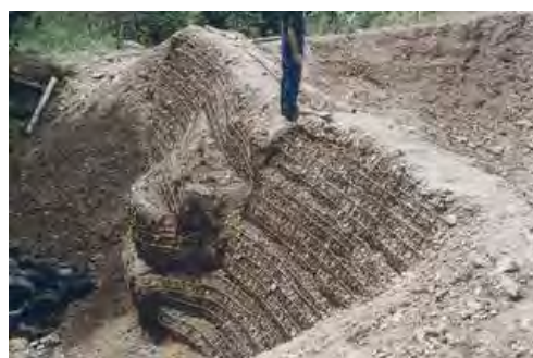
Figure 8. Rockfall protection embankment after impact evidencing relative displacement between soil layers associated with horizontal reinforcement (from Peila et al., 2007).
