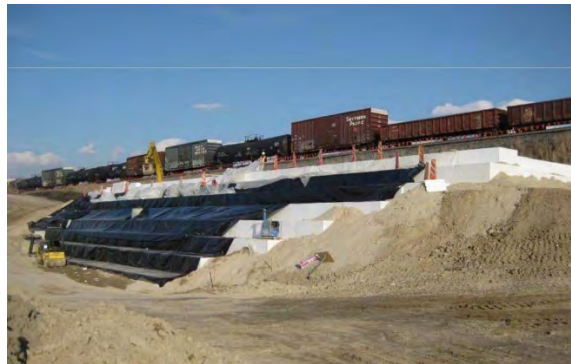
Figure 8. Geomembrane over Geofoam in Railway application. Salt Lake City UT USA. Source: University of Utah
