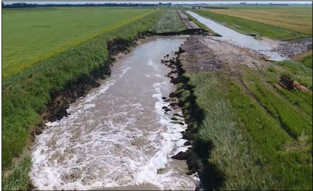
Figure 1. Channel Erosion prior to remediation.
