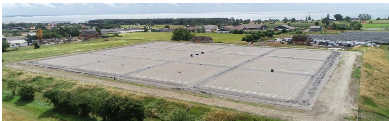
Figure 10. Insulated floating cover on a hot water thermal pit. Marstal, Denmark. (Image: AalborgCSP, 2019).
