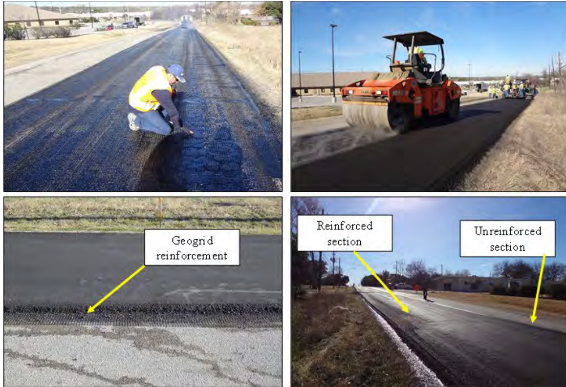
Figure 5. Final paving work at the geosynthetic-reinforced section.
