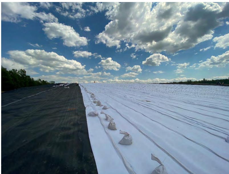
Figure 12. Infiltrated rainwater drainage geocomposite
