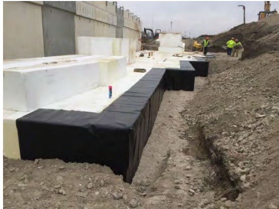
Figure 6. Geomembrane over Geofoam edges. I75 Toledo OH USA
