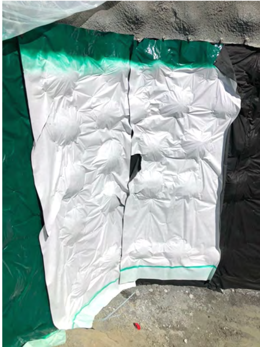
Figure 3. Conforming the Geotextile into A Corner
