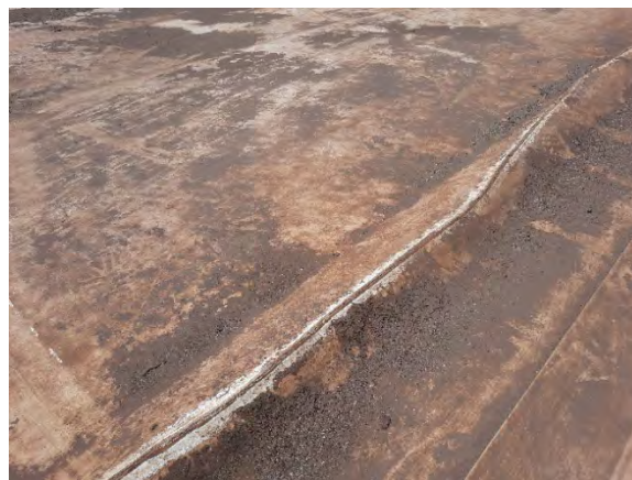
Figures 12 & 13. Surface cracks found in the RPP liner material folds and creases
