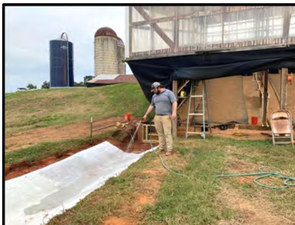
Figure 13. Spraying Water to Hydrate Product
