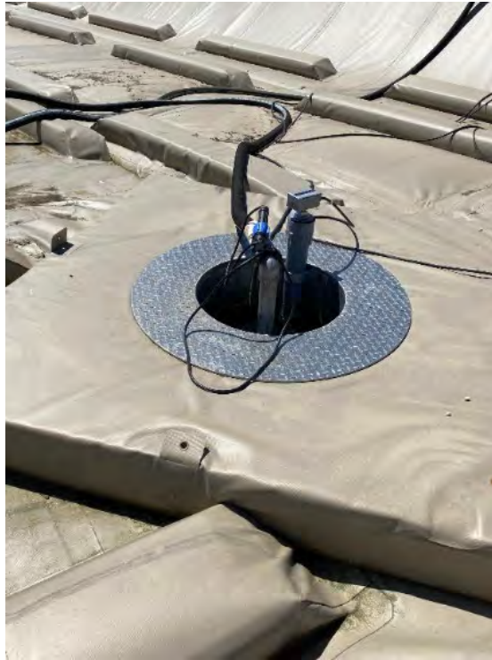
Figure 4 – Rainwater Removal System
