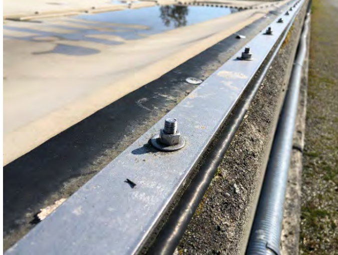
Figure 10 Floating cover mechanical anchorage at parapet wall
