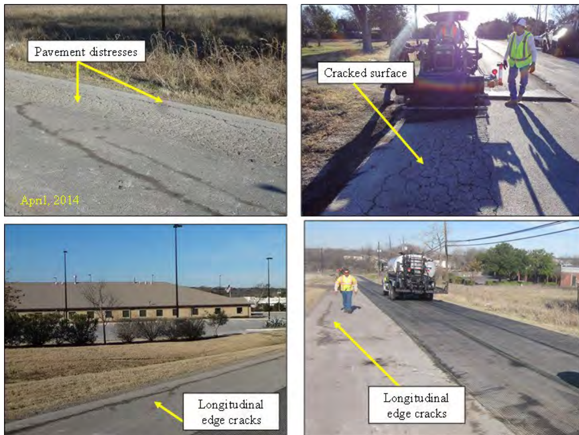
Figure 3. Distresses in the Pre-existing Roadway: April 2014.
