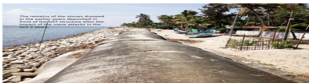
Figure 9. Geosynthetic Tubes as Seawalls for Coastal Protection, at Vypeen Reach. (Source: KID)
