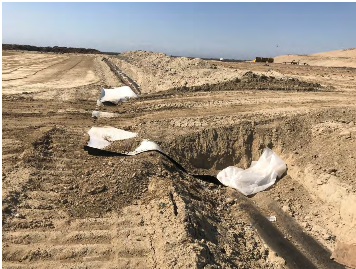
Figure 2. Method of Electrically Isolating Access Roads
