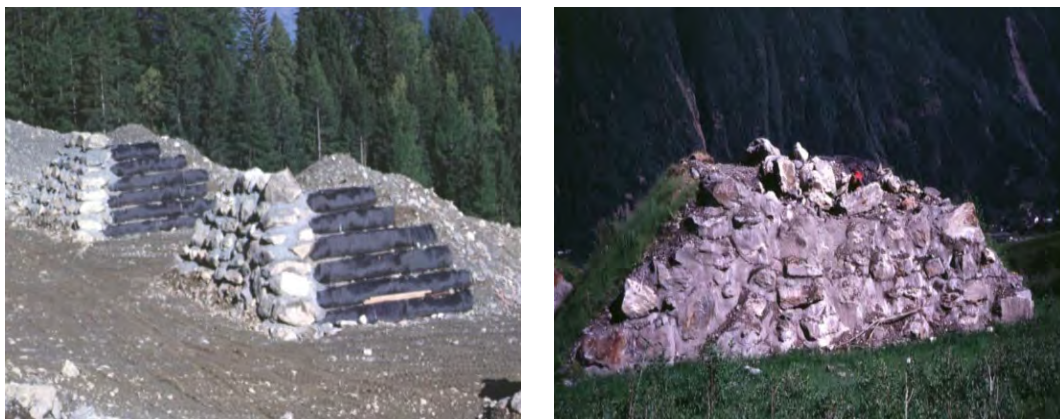
Figure 7. Avalanche breaking mound after completion (left) and after partial destruction (right). Location: Taconnaz, France. (J.M. Tacnet, INRAE).
