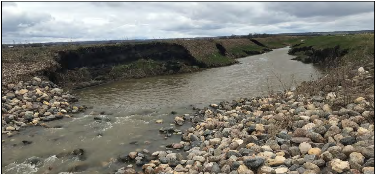
Figure 12. Unreinforced Section showing erosion and geotechnical failures after storm event - Upstream Section (05/2022)
