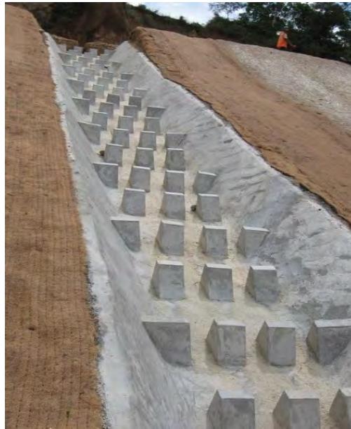
Figure 1. Energy dissipaters incorporated as part of a concrete-filled geocell mine channel, Peru
