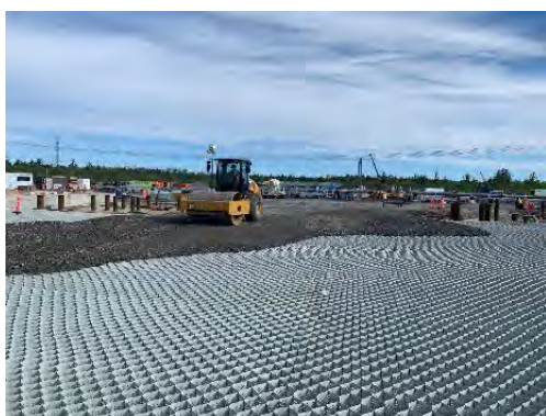
Figure 13. Top layer geocell being built
