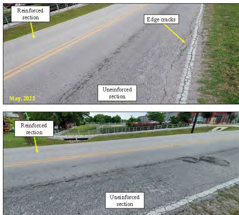
Figure 7. View of road condition of a geogrid-reinforced section (left) and control section (right) showing edge cracks in the unreinforced section.
