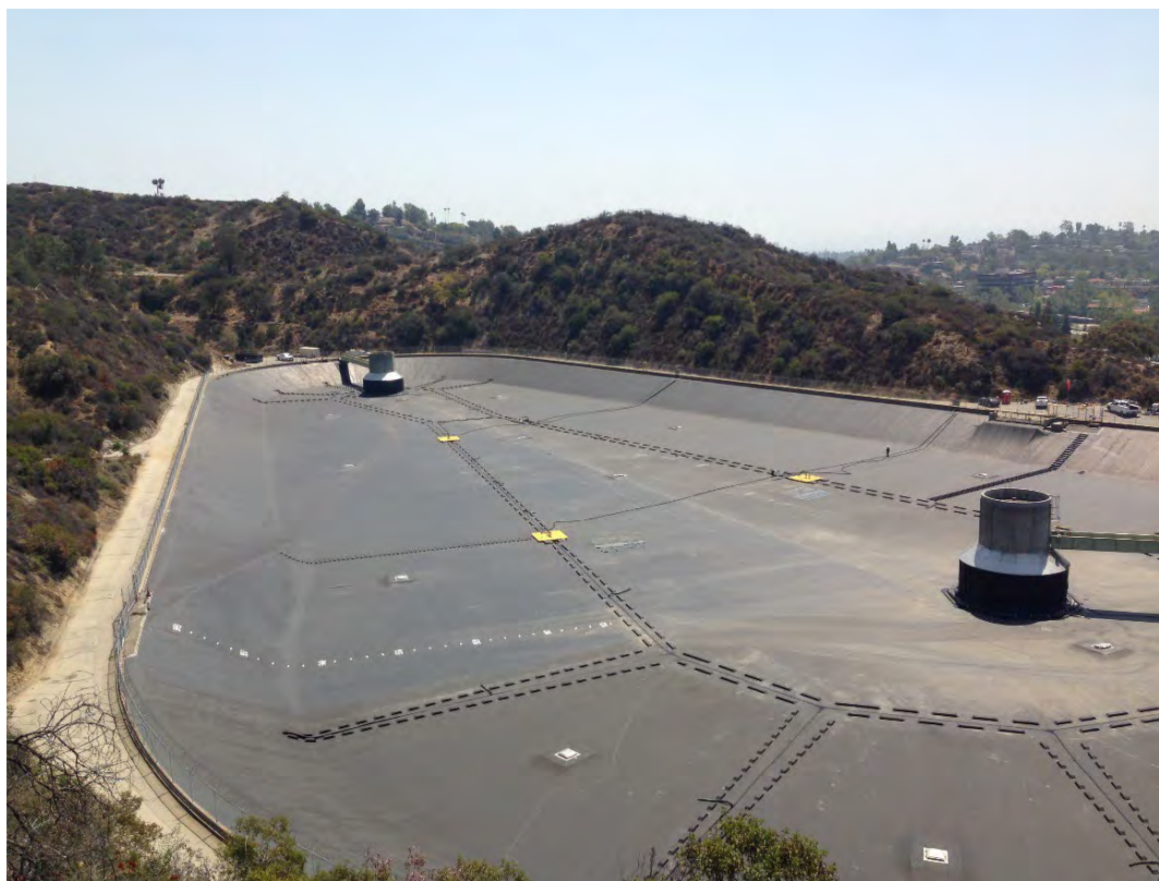
Figure 1. 350,000 ft 2 Floating Cover Eagle Rock Reservoir, CA USA
