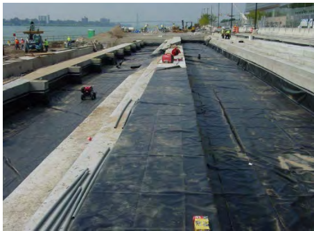
Figure 11. Geomembrane deployed over Geofoam.
