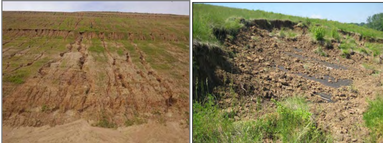
Figure 7. (a) Poor vegetation and erosion gullies on traditional soil cover (b) Veneer slope failure of traditional soil cover (Maier, 2012).
