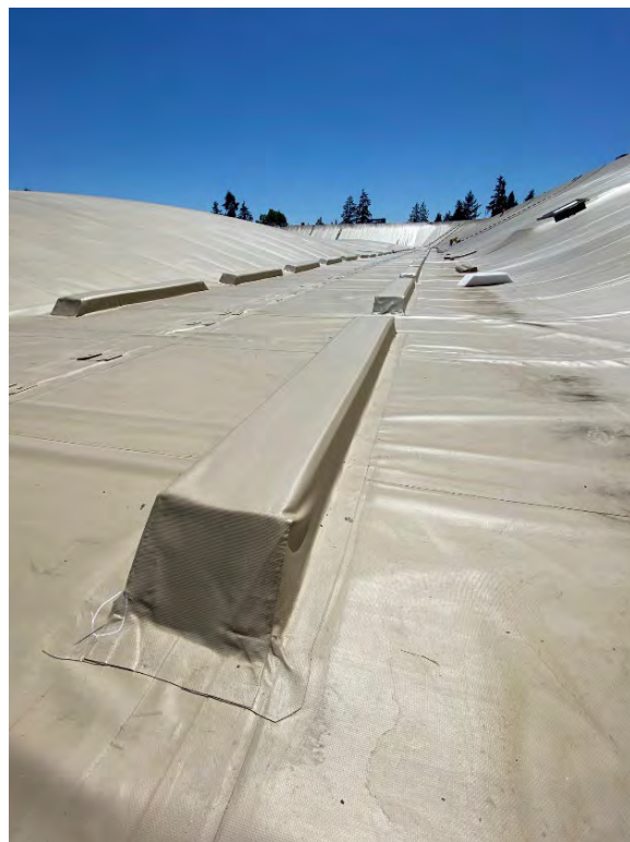
Figure 7 and 8. Inflation via access hatch and west cell cover undergoing inflation inspection
