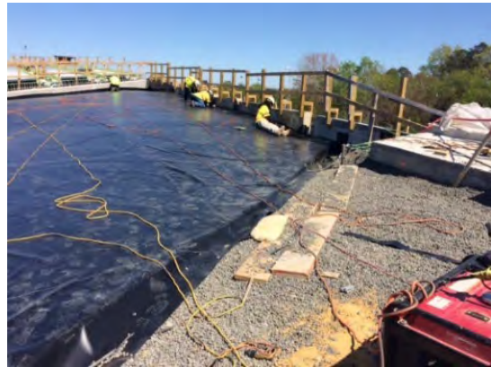
Figure 7. Geomembrane completion over Geofoam. Norfolk VA USA
