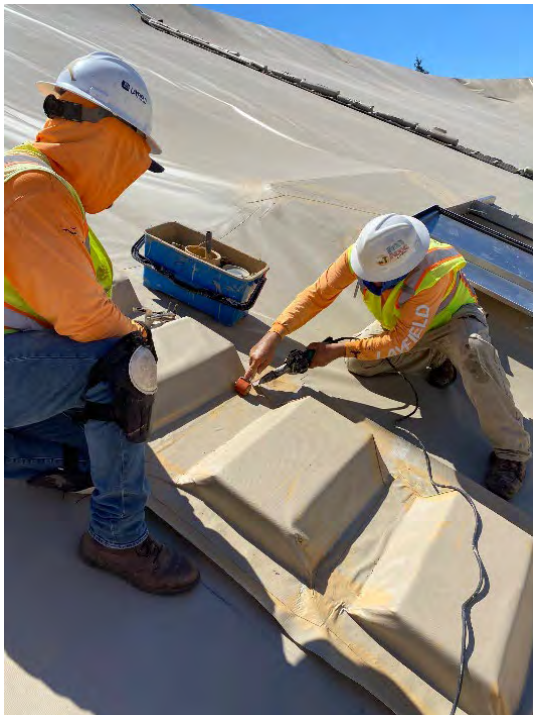
Figure 5 and 6. Crews installing fabricated entry stairways and welding floating cover seams
