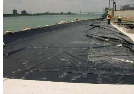
Figure 10. Geomembrane Installation over Geofoam.
