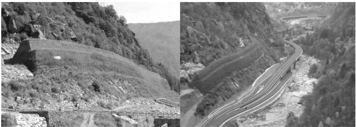
Figure 1. Huge rockfall protection embankment protecting the Simplon road, in Varzo, Italy (Rimoldi et al., 2008).
