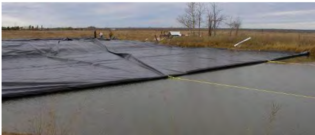
Figure 8. Floating cover being pulled into place with rope and reinforced leading edge.
