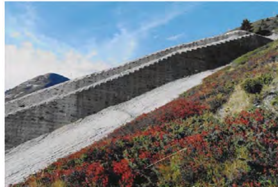
Figure 4. Snow avalanche deflecting dam in Belle-Plagne, France (Coulon and Bruhier, 2006).
