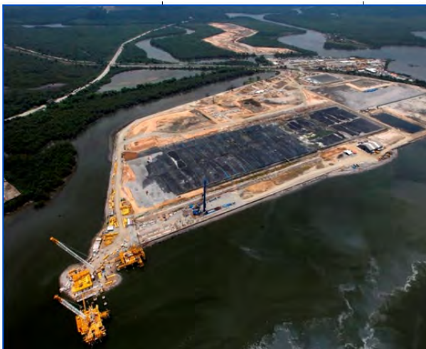
Figure 18. Covering the geotextile tube containers
