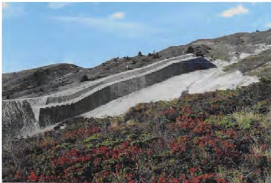
Figure 4. Snow avalanche deflecting dam in Belle-Plagne, France (Coulon and Bruhier, 2006).
