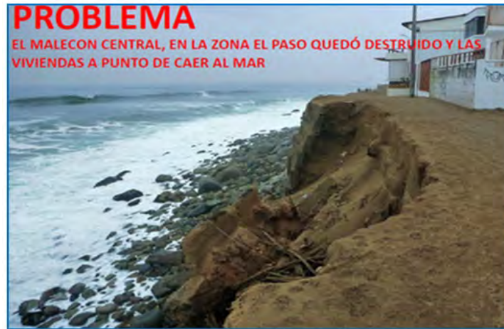
Figure 21. Collapsing shoreline required immediate protection
