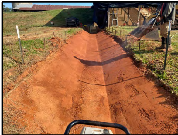
Figure 11. Trapezoidal Channel Prepared
