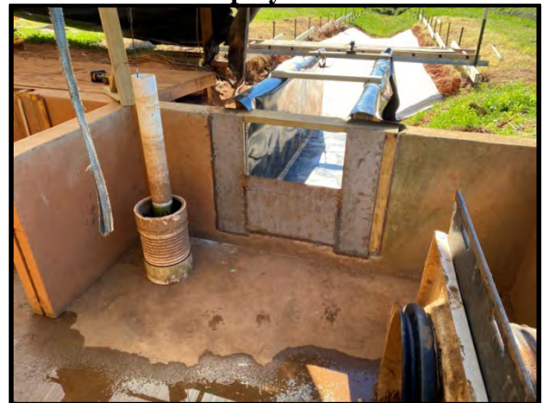
Figure 14. Upstream Sharp Crested Weir
