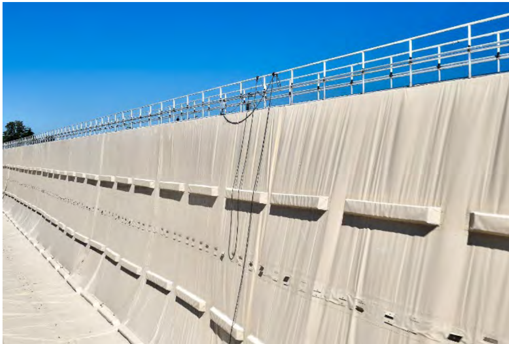
Figure 2. Installation underway of double trough system on 28-foot divider wall on west cell
