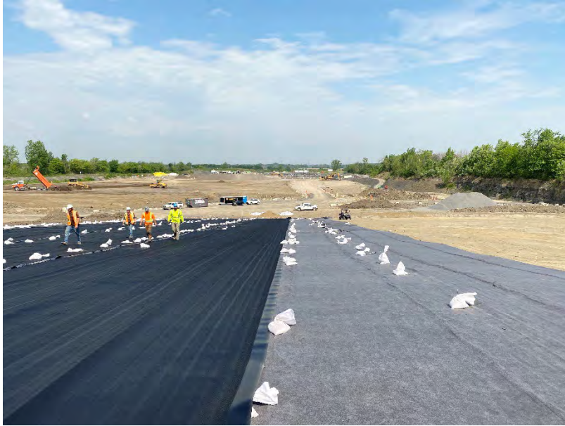
Figure 11. Installation of the geomembrane on the geocomposite
