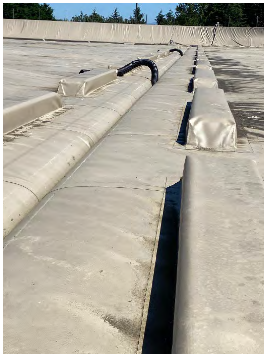
Figure 9. East cell trough & floats in service
