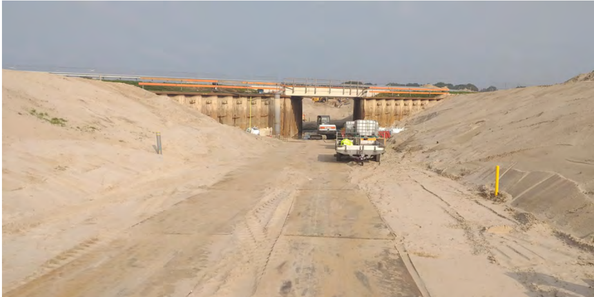
Figure 5. Ramp after backfilling and dewatering
