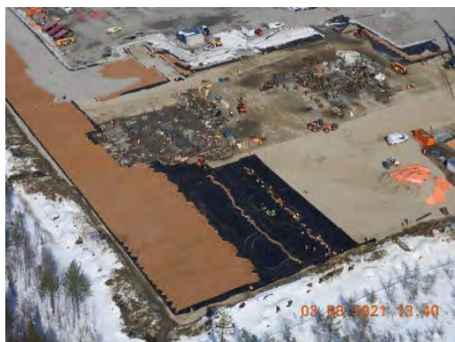
Figure 12. Progress of 3 layers of geocell through winter
