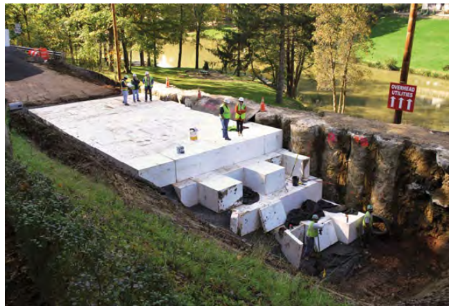
Figure 1. Typical Geofoam Application. Source: EPS Alliance
