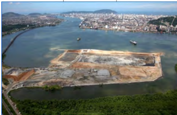
Figure 16. Partially constructed perimeter dike
