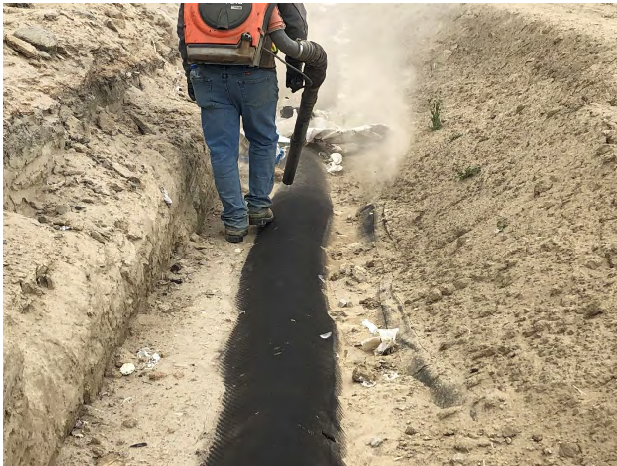
Figure 3. Backpack Leaf Blower Used to Dry out the Geocomposite in the Perimeter Isolation Gap.
