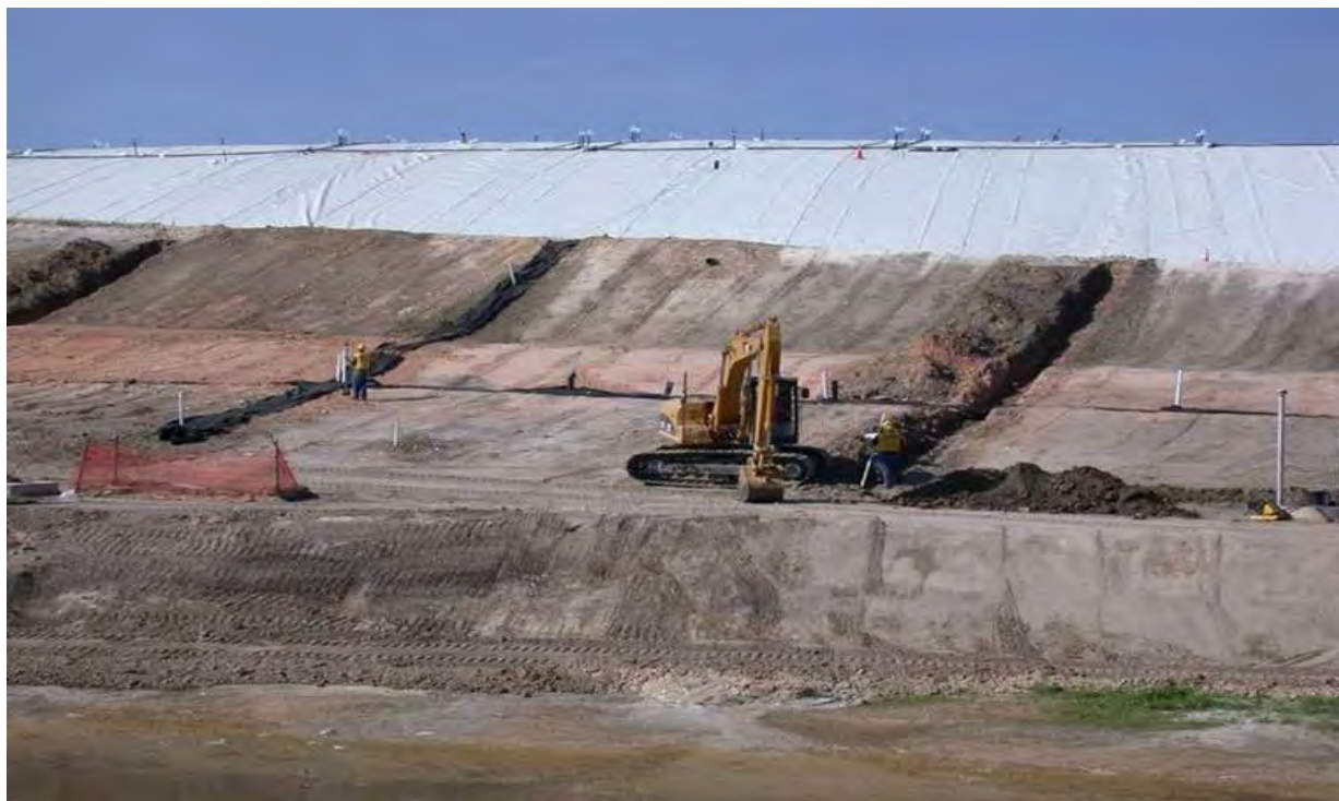
Figure 4 – EGC Anchor Trench Construction
