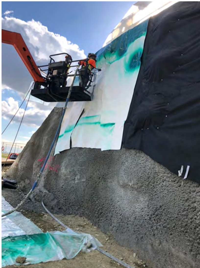
Figure 2. Applying Polyurea to the Conductive Geotextile
