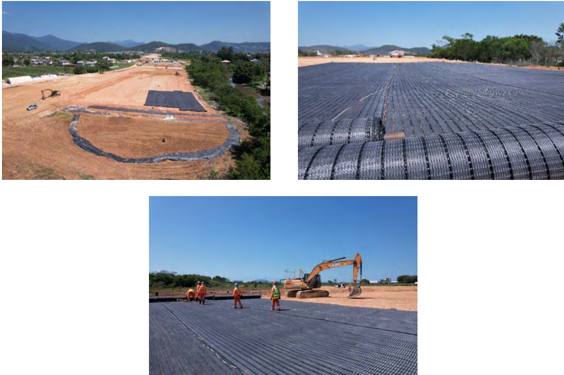
Figure 8 – Installation of the 1750 kN/m Geogrid
