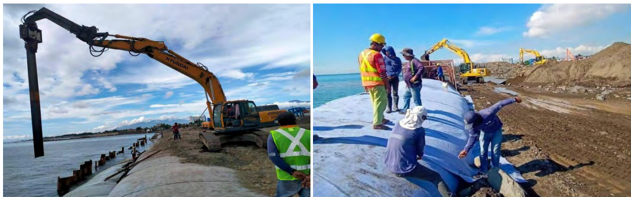
Figure 11. Installation of sheet piles for toe protection and geotextile protection layer
