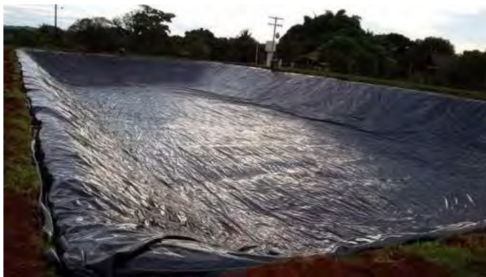
Figure 6: Rectangular tank coated with PVC geomembrane
