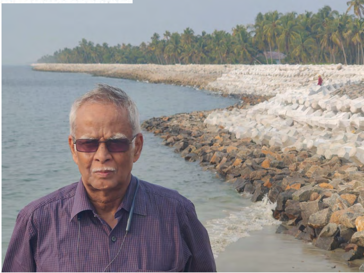
Figure 5. A Rubble-Mount Seawall with Concrete Tetrapod as Armour Layer Reach Under Construction at Challam Coast (Nov 2022). (Source: KID 2022)
