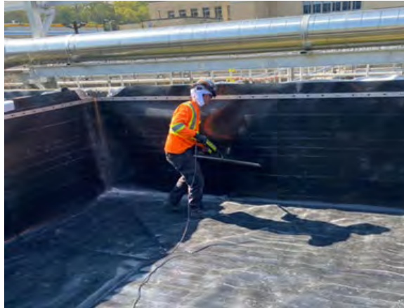
Figure 5. Technician performing arc testing on the primary liner
