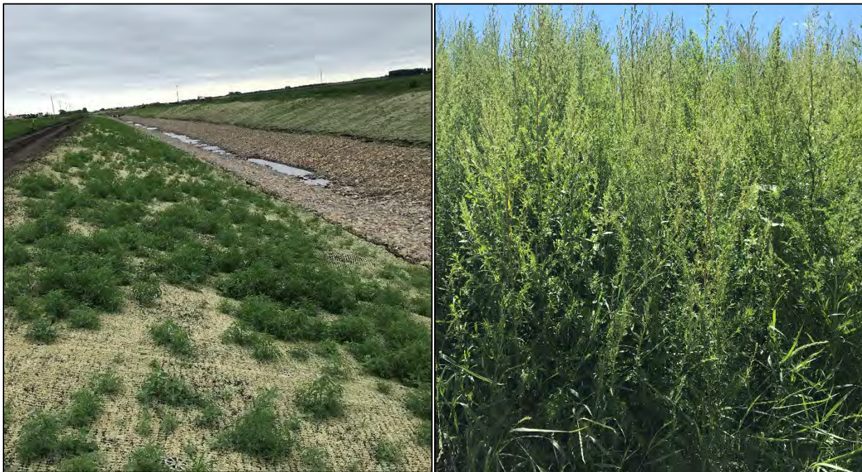
Figure 8. Hydroseeded EEAS (06/2018 - Left) and Vegetation beginning to Establish (07/2018 – Right)
