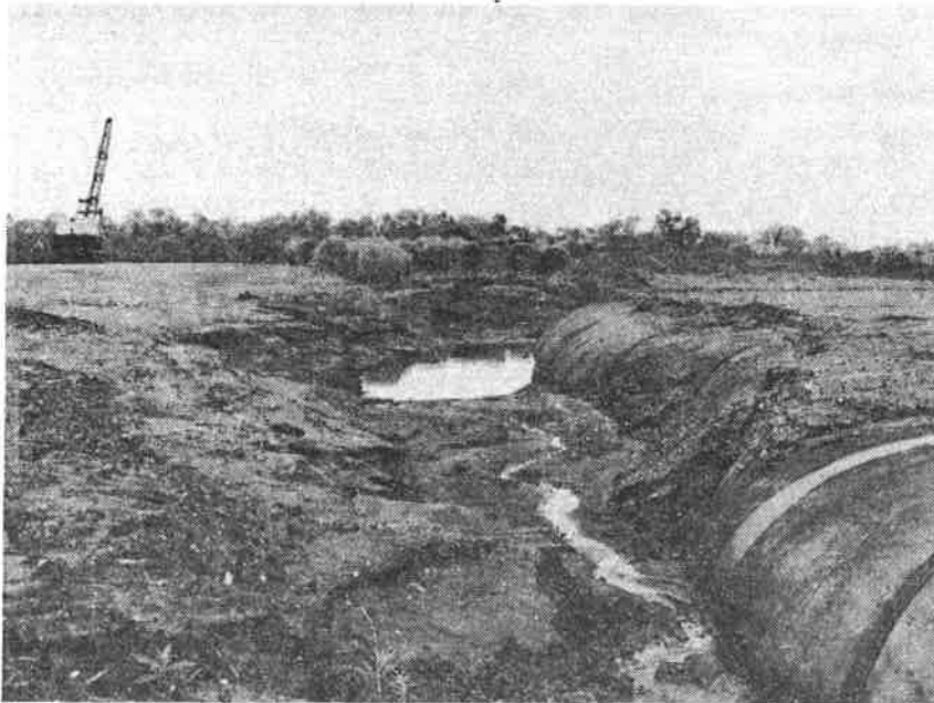
FIGURE 5. VIEW OF THE SITE SHOWING GEOTEXTILE BUBBLE
