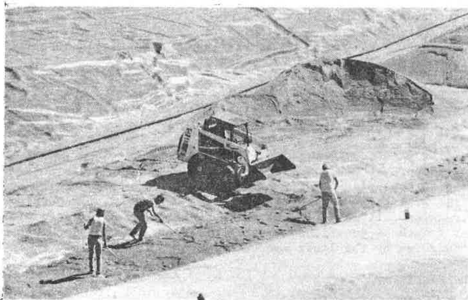
Figure 7. Front-end loader used to transport drain material to secondary leak detection pipe trenches.
