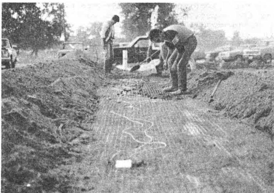
Photo 3 : Alignment of Strain Gauges for Geogrids
