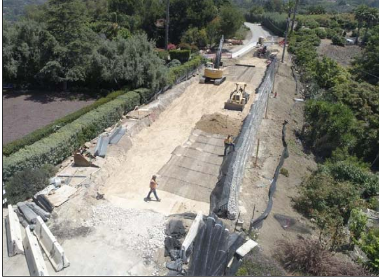
3 FT of engineered fill is brought on top of TDA, to bridge over material and provide stable base for structure section. Tensar UX1100 (or equal) specified. TerraGrid U350 Used.
