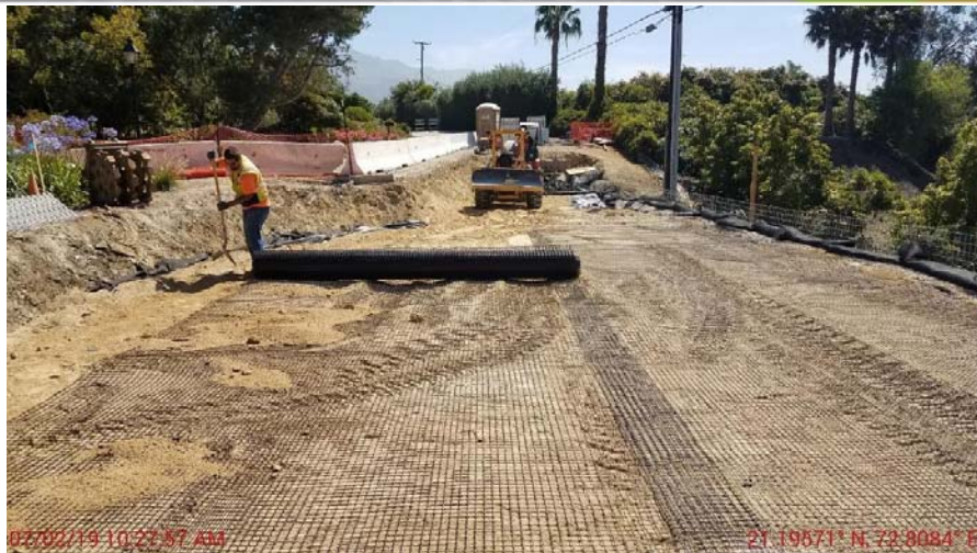
2 layers of biaxial geosynthetic reinforcement are placed within engineered fill to full width of excavation. Tensar BX1500 (or equal) was specified. TerraGrid SX3030 used.
