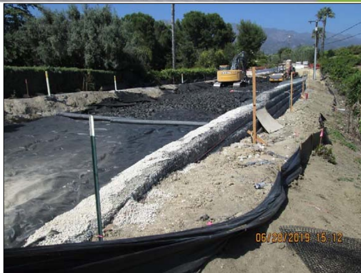
Subgrade Enhancement Geotextile ( TerraTex HPG-16ca ) is placed on top of the TDA prior to engineered fill placement.
