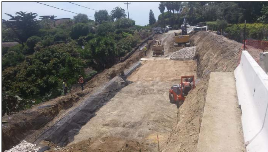
Placement of engineered fill, first level of MS-TDA Wall facing, stone fill, and Geosynthetic reinforcement.
