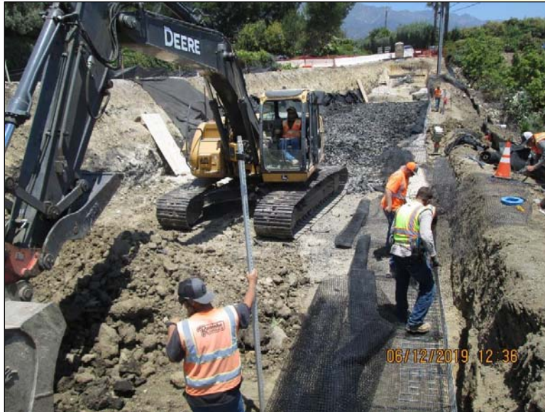
Contractor must maintain multiple operations at same time to progress the work.
