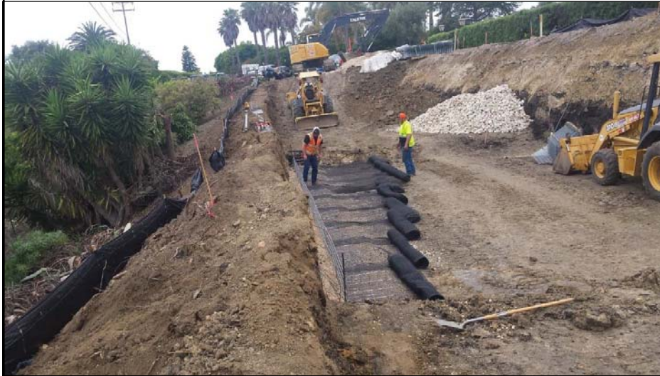
Placing the first level of MSE Wall welded wire facing on engineered fill, and placement of Tensor UX1100 (or equal) uniaxial geosynthetic reinforcement.
