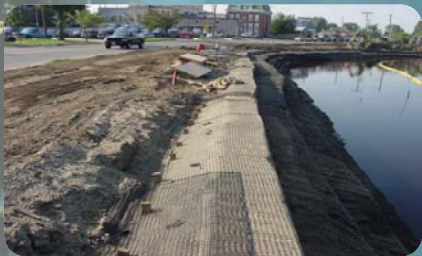
Secured geogrid & geotextile
