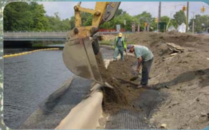
Geogrid, batter board & geotextile
