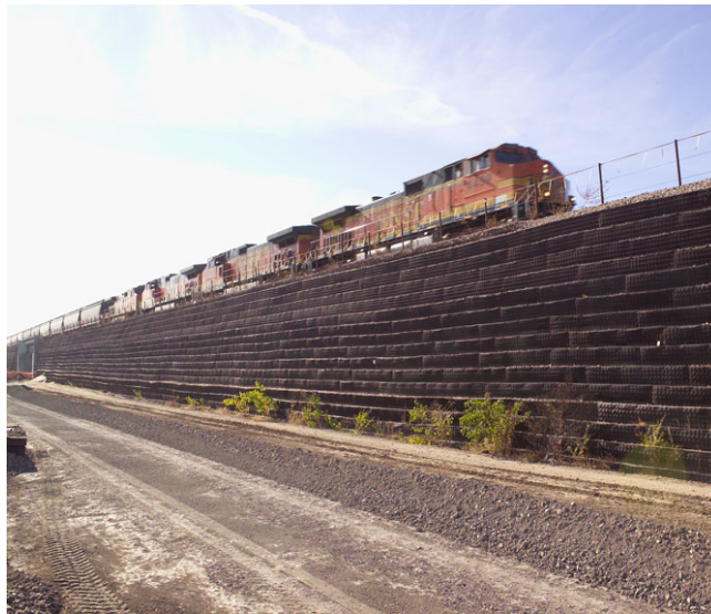
Figure 1. WWM MSE wall in a railway application
