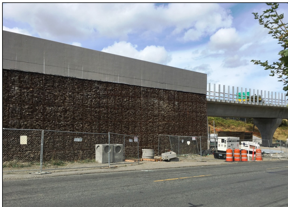
Figure 2. Finished Wall Photo
