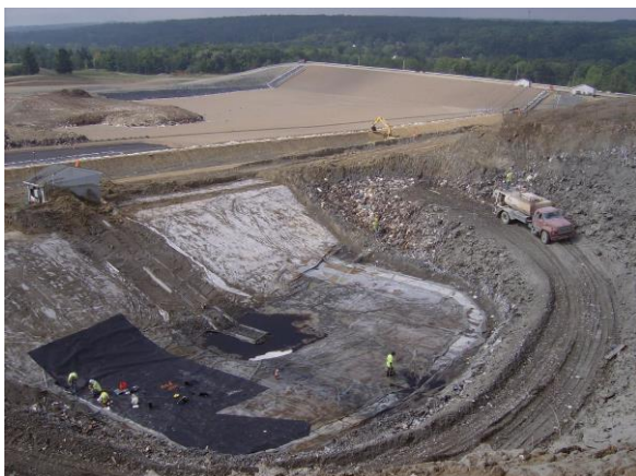
Fig 1- Overview Photograph of Site #1
