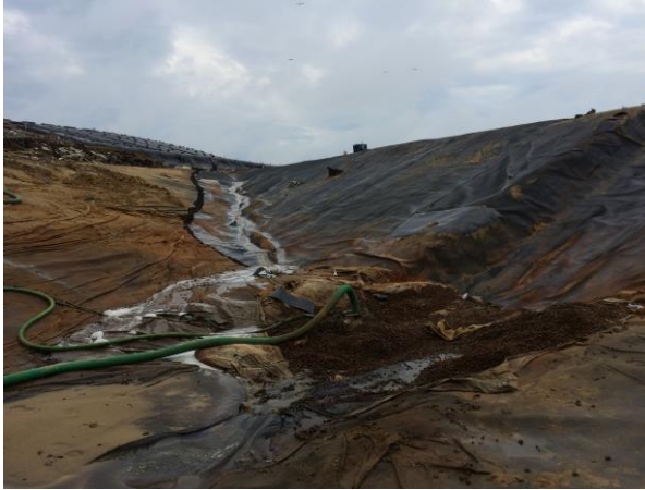
Fig 3- Overview Photograph of Site #2
