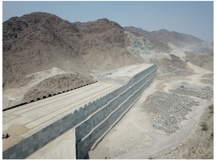
Figure 1. 43 M high Geosynthetic Strip MSE Wall in construction.
