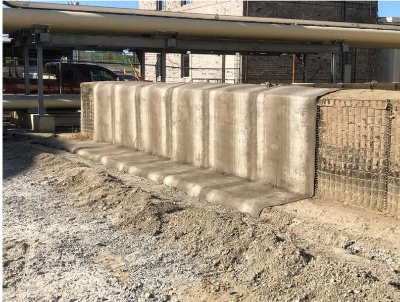
Similarly, soil/sand filled wire baskets (aka gabions) have long been used as shoreline protection and flood control and widely utilized by military engineers as rapid deployment defenses not solely for flood control but as semi-permanent blast walls against explosions or small arms. In some of these military applications, the gabions, once placed and filled, have been further armored by various coverings, of which GCCMs have excelled.
