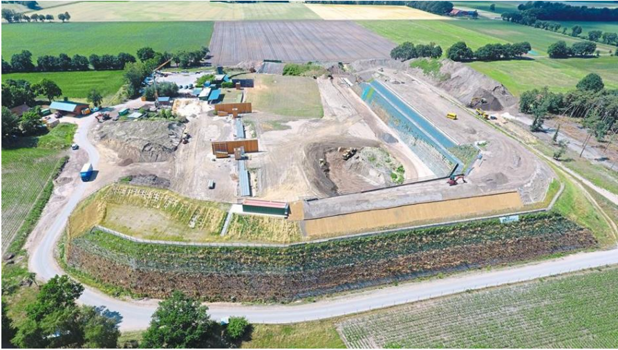
Figure 1. Bird’s view of the noise and bullet barrier in Hopsten
