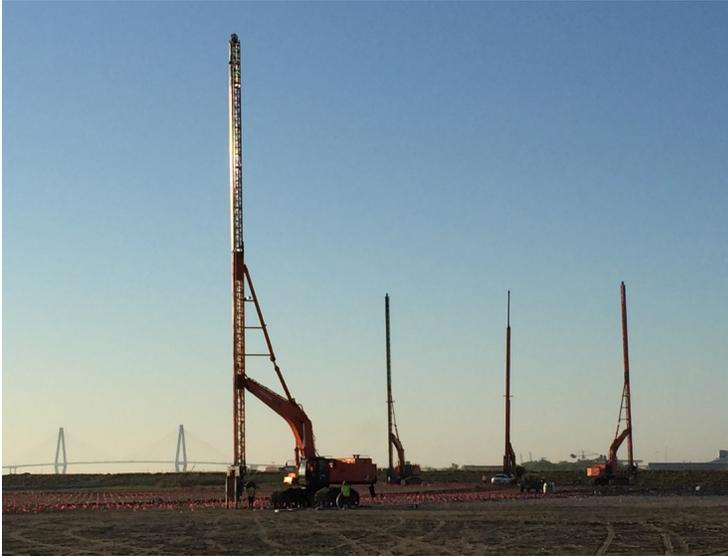
**Figure 2. Installation of prefabricated vertical drains.**
