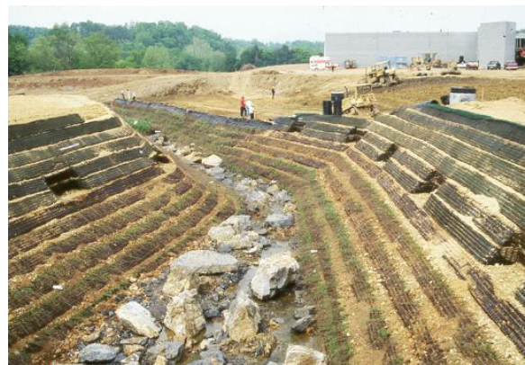
Figure 2 – Immediately After Construction
