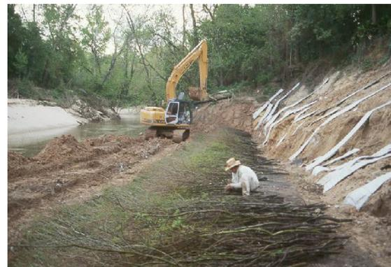
**Figure 2. Installing live cut branches**
