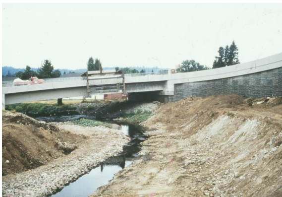
Figure 5. Original 1993 design for riprap
