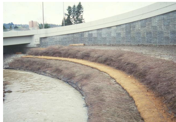
Figure 6. 2 weeks post construction 1994
