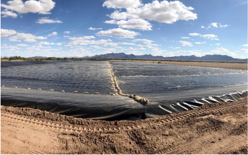
RPP Geomembrane panels secured in perimeter anchor trench.
