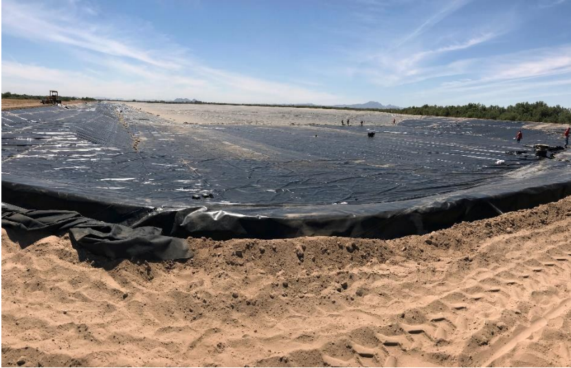
Anchor trench preparation and fill work to secure the RPP liner.
