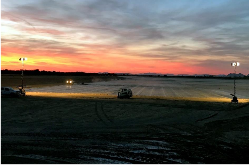
Evening installation of RPP Geomembrane prefabricated panels.
