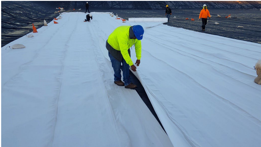
Figure 3. Draintube Conductive installation
