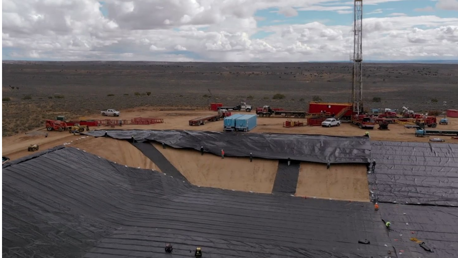
Figure 2. RPE geomembrane installation
