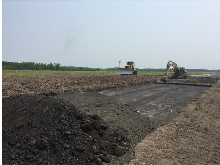
Photo 2: Processed R.A.P. Used for Granular Layer at General Aviation Airport
