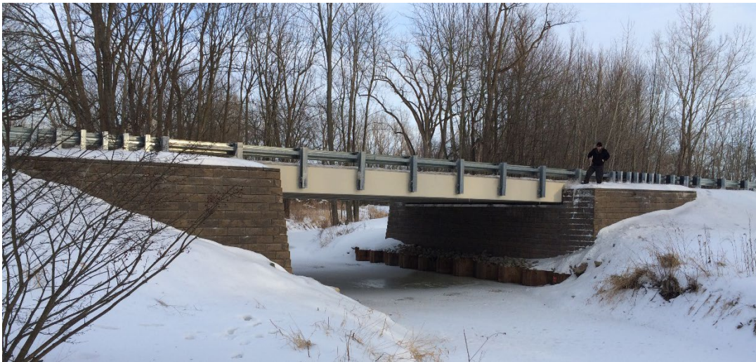
Figure 1. GRS IBS bridge replacement on Kefer Highway in Ionia County, MI Source: FHWA
