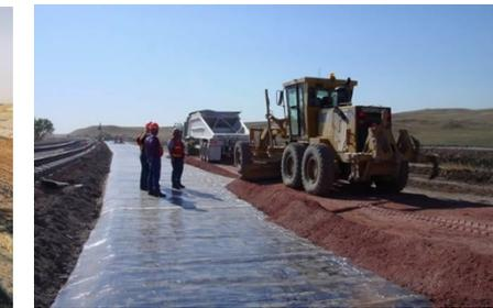
**Figure 7. Sub-Ballast Placement**
