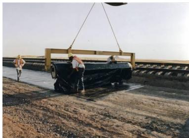
**Figure 6. Placing BGM**
