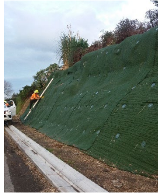
Installed HPTRM (prior to vegetation)
