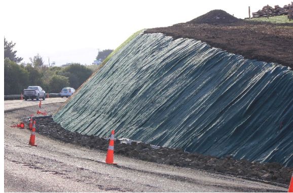
Installed TRM (prior to vegetation)
