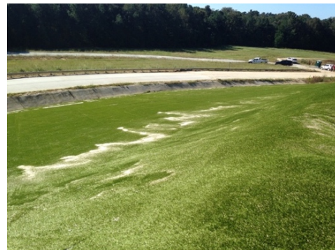
(b). Engineered Turf Cover Area
