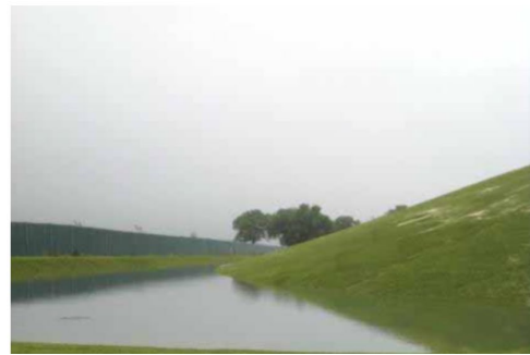
(b). After Closure with Engineered Turf Cover
