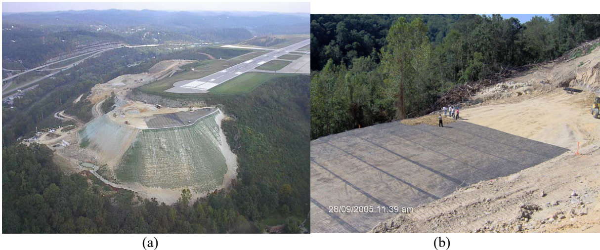
Figure 1: Photograph of RSS Nearing Completion (a) and During Construction (b)
