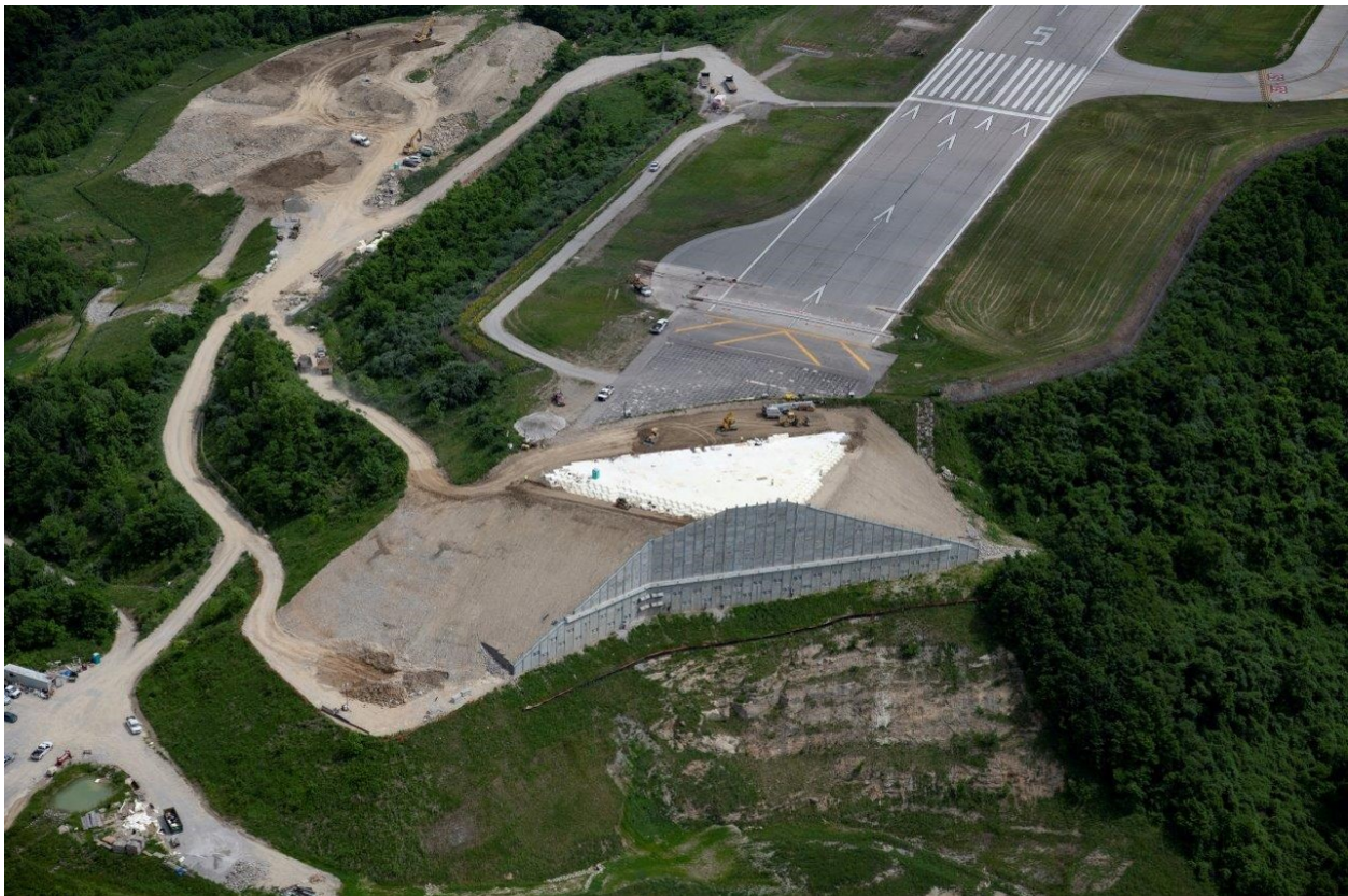
Figure 1. Aerial view of EPS backfilled retaining wall at Yeager Airport
