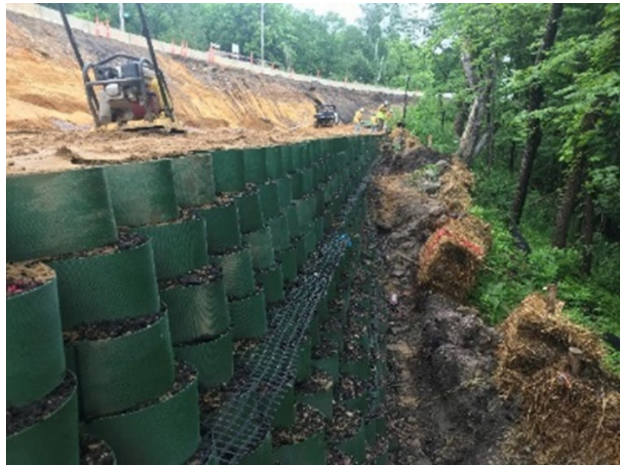
Figure No. 3 – 1H:2.75V RSS with stacked Geocell face Figure No. 4 – 30 ft tall 1H:2.75V RSS with vegetated Geocell face
