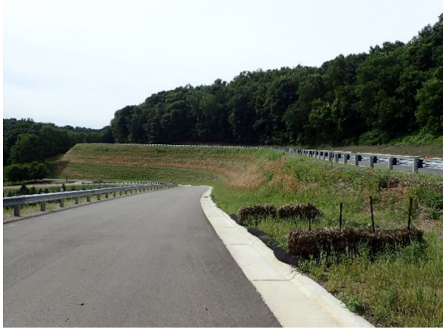
Figure No. 2 – 30 ft tall 1H:1V upper RSS tier as shown on Figure No. 1
