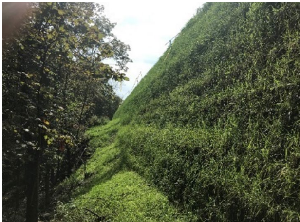
Figure No. 3 – 1H:2.75V RSS with stacked Geocell face Figure No. 4 – 30 ft tall 1H:2.75V RSS with vegetated Geocell face
