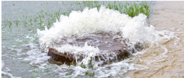
Figure 1. Sanitary Sewer Overflow
