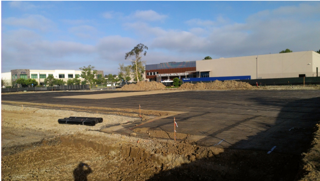
Figure 3. Geogrid Layers within Compacted Fill
