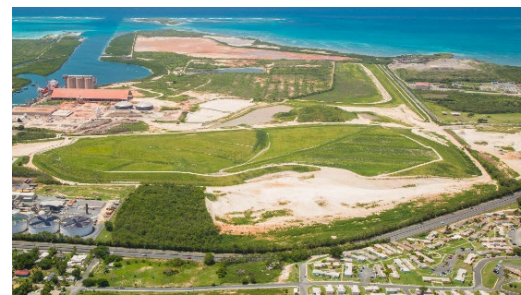
Photo 5. Area A Site Post Remediation
