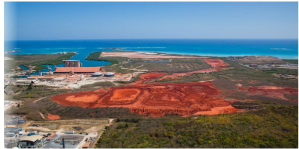
Photo 1. BRDA Site Before Remediation
